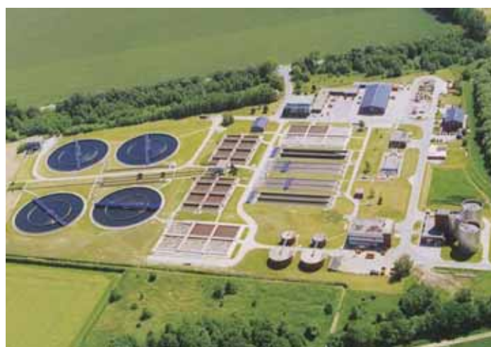
Large wastewater treatment plant in Germany
